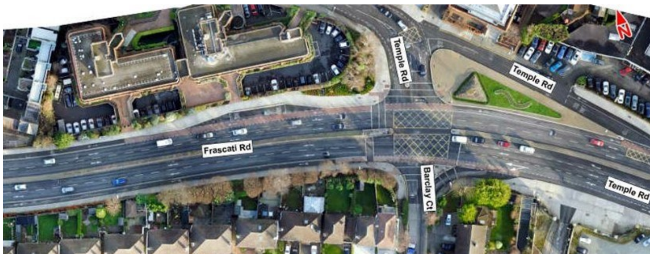
Image 6.5: N31 Frascati Road / L1011 Temple Road / N31 Temple Road / Barclay Court Junction
