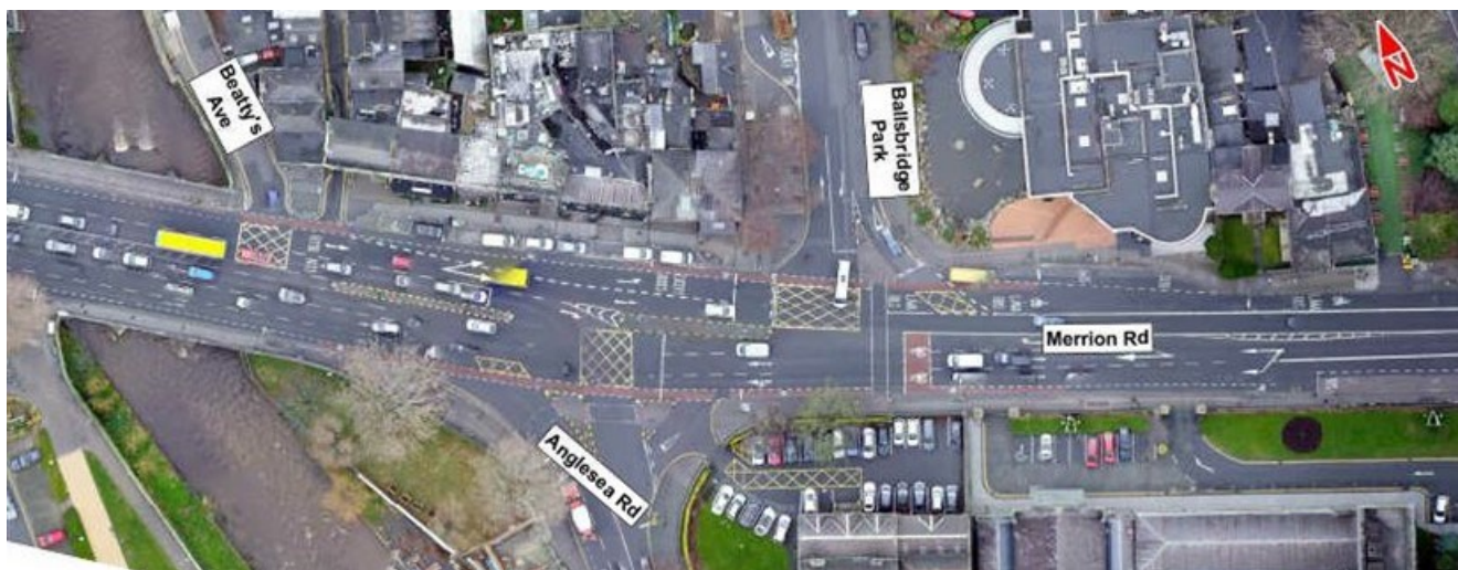
Image 6.33: R118 Merrion Road / Ballsbridge Park / Anglesea Road Junction
