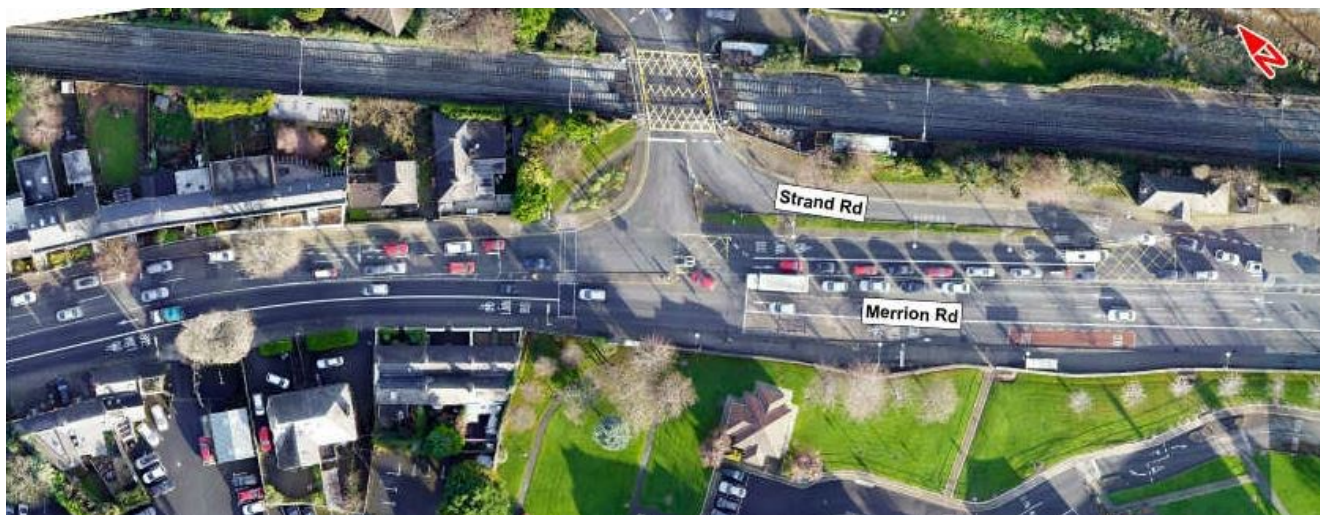
Image 6.21: R118 Merrion Road / R131 Strand Road Junction
