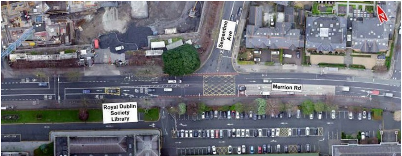
Image 6.32: R118 Merrion Road / Serpentine Avenue Junction
