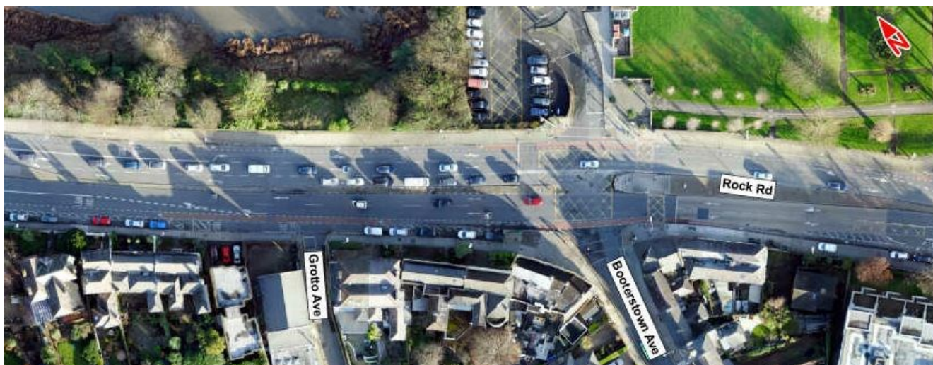
Image 6.15: R118 Rock Road / Booterstown Avenue Junction / Booterstown DART Station Car Park
