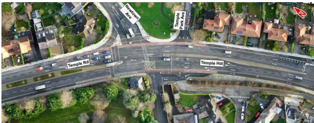
Image 6.3: R113 Temple Hill / Temple Road / Newtown Avenue Junction
