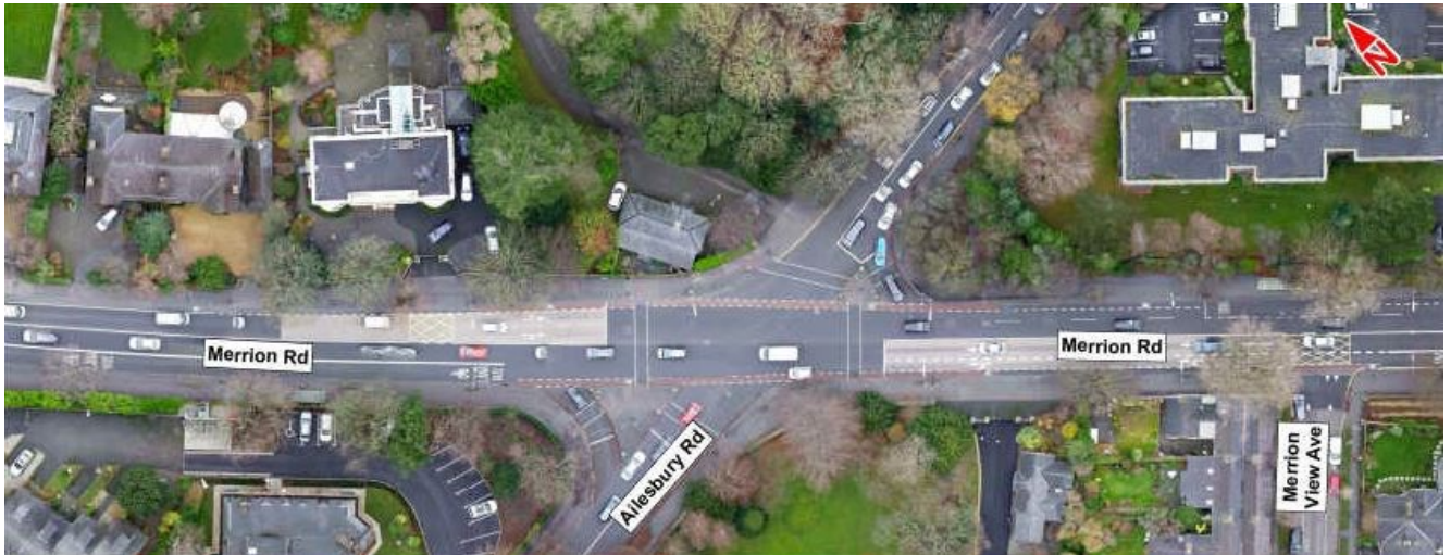
Image 6.26: R118 Merrion Road / Ailesbury Road Junction
