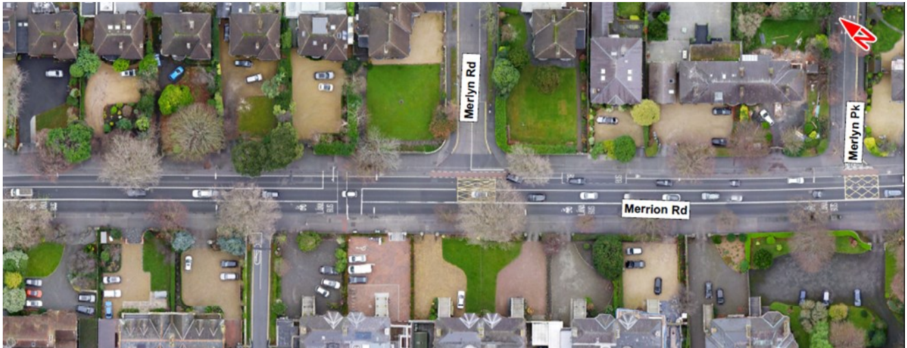
Image 6.28: R118 Merrion Road / Merrion Road Junction
