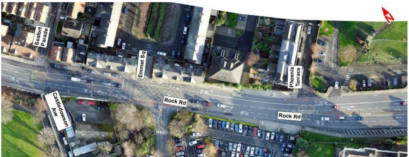
Image 6.12: Rock Road / Phoenix Terrace Junction
