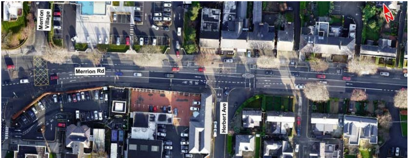
Image 6.22: R118 Merrion Road / Herbert Avenue Junction
