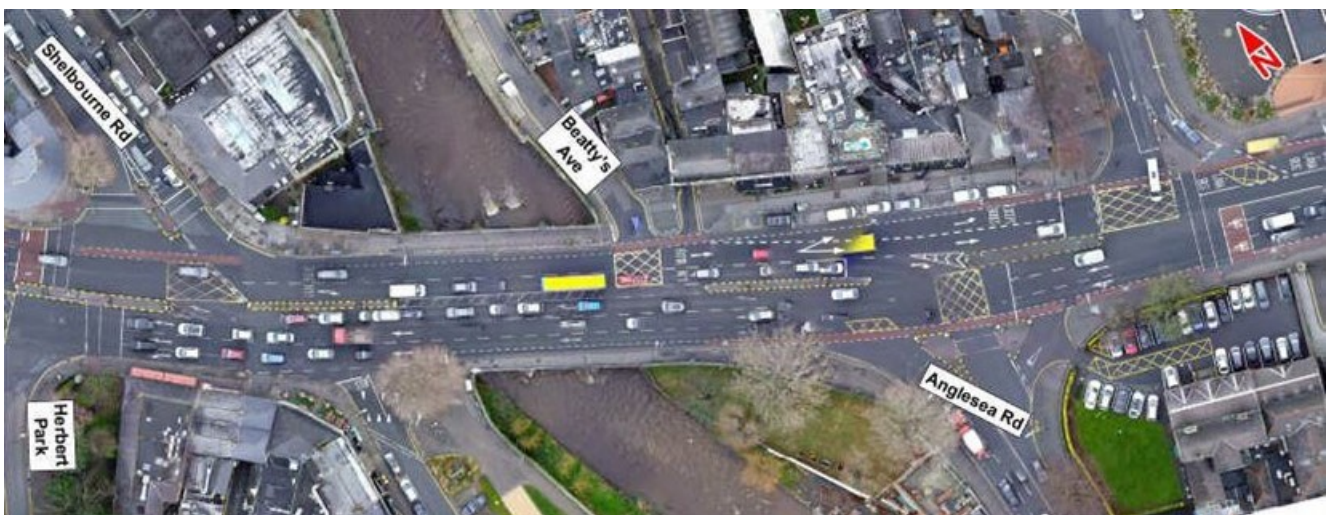
Image 6.34: R118 Merrion Road / Beatty's Avenue Junction
