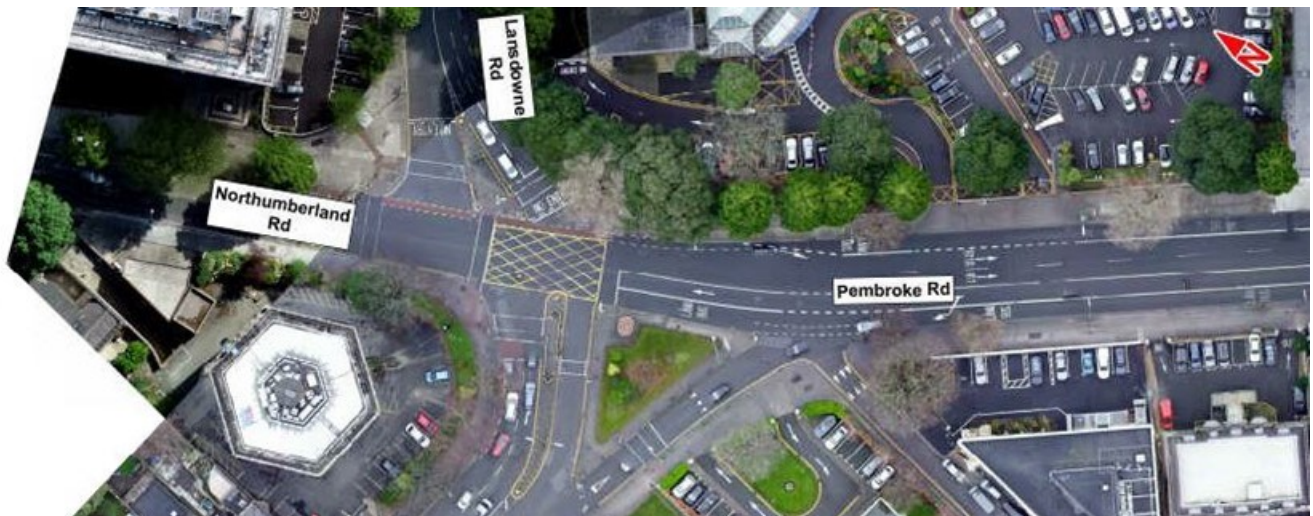
Image 6.37: R118 Northumberland Road / Lansdowne Road / R118 Pembroke Road / R816 Pembroke Road Junction
